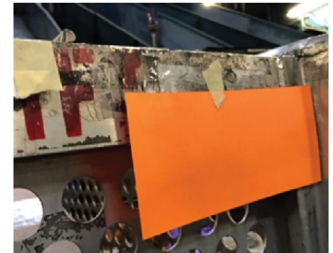
Figure 5. Examples of Missing or Deficient Label Placards
