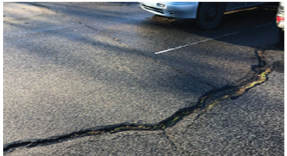
Figure 12. Cracked Asphalt
