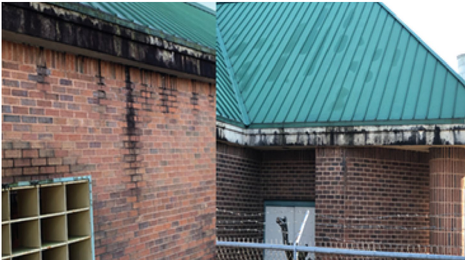
Figure 11. Dirty Exterior Trim at Rear and Sides of Building
