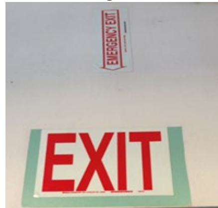
Figure 10. Exit Signs Not Illuminated
