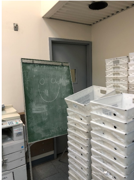
Figure 13. Blocked Inspection Door
