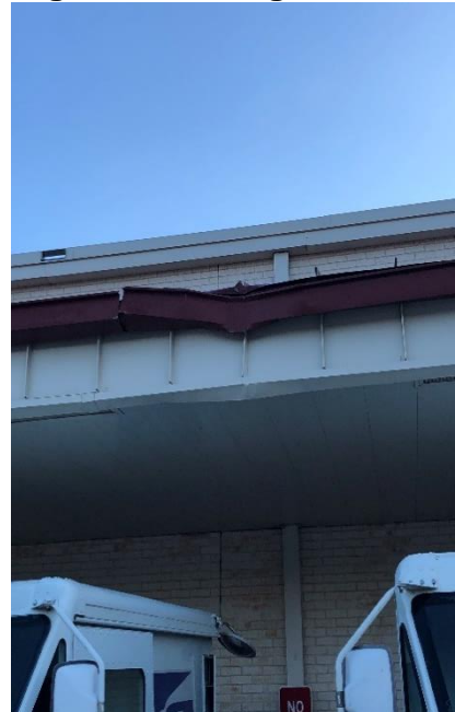
Figure 5. Damaged Gutter
