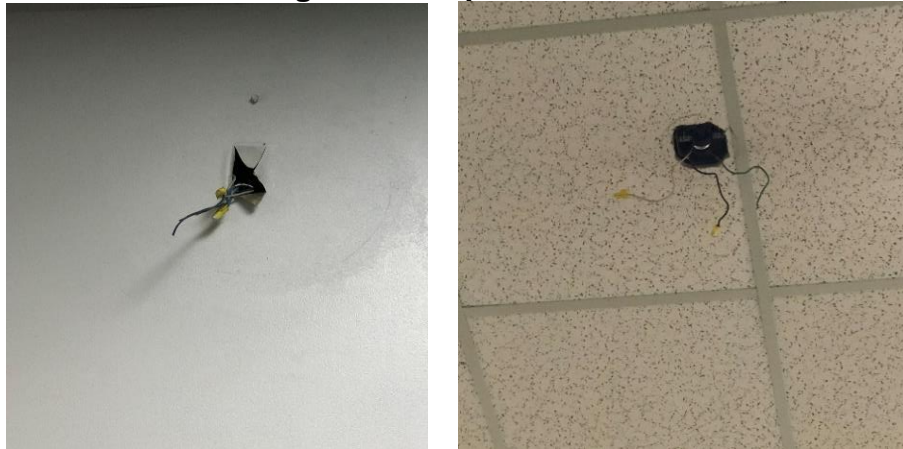
Figure 14. Exposed Wires
