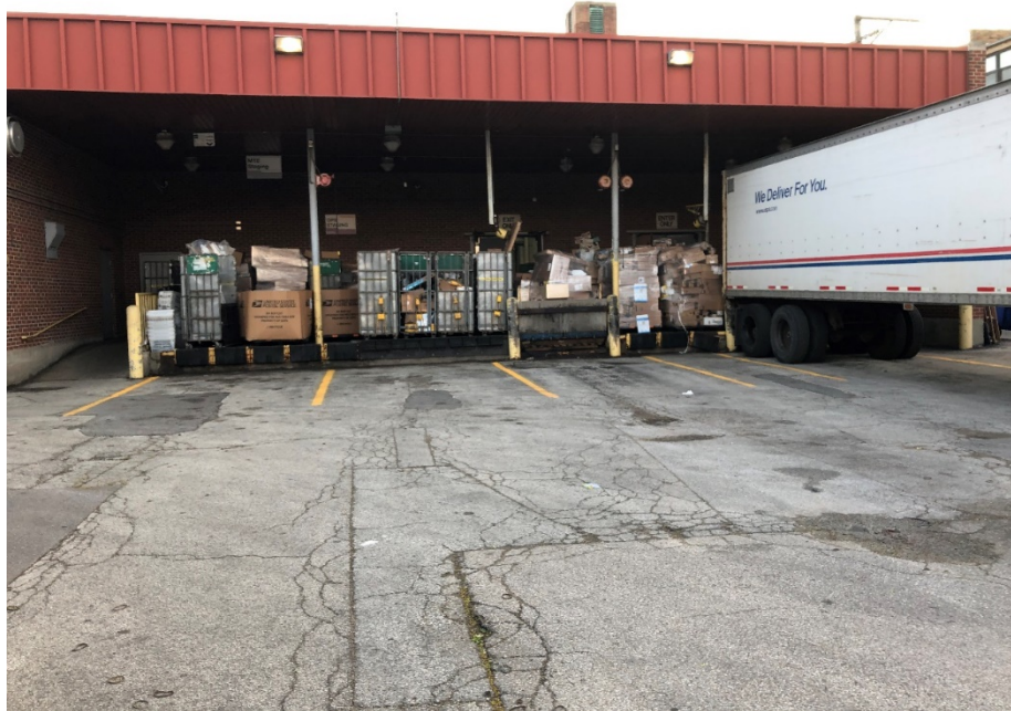
Source: OIG photographs taken during fieldwork at Henry McGee Station on 6/10/2020.
