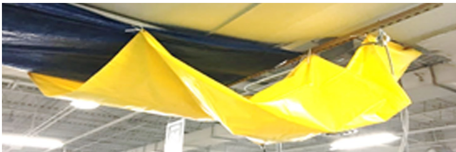
Ceiling leakage.
