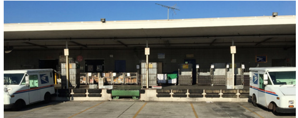
Figure 9. Unattended Mail Secured by Fence and Gate
