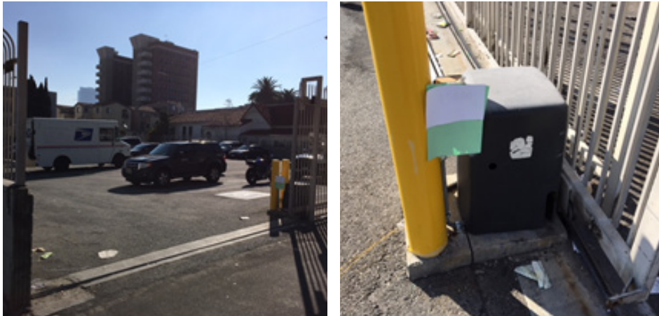
Figures 7 and 8. Security Gate Held Open by Paper Over the Sensor
