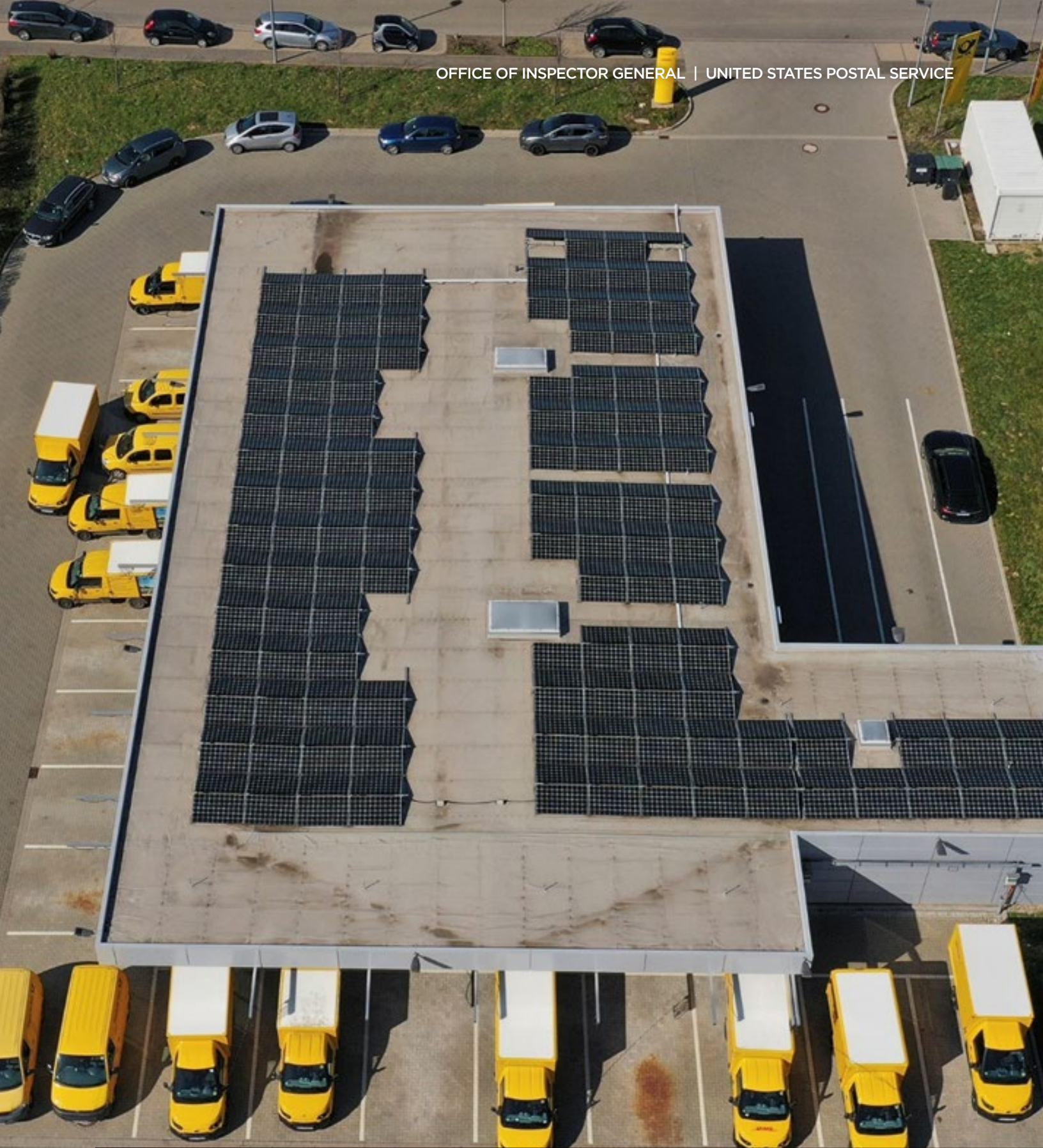
Rooftop solar panels provide renewable energy to this Deutsche Post DHL Group facility in Wachtberg, Germany.
