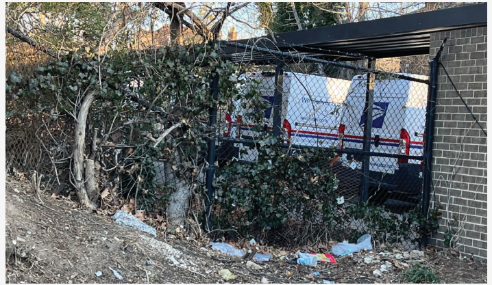
Figure 6: Trash and Overgrown Foliage
